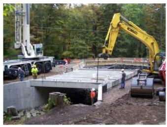
Photo: Saugerties contractor Advanced Enterprise Concrete & Excavation, Inc. worked for the Town of Olive to construct a new stream crossing with NYC funding, managed and administered by CCEUC for the Ashokan Watershed Stream Management Program. The previous culvert was under-sized and constricted stream flows. The new bridge passes the 1:100-year return frequency storm flow.
